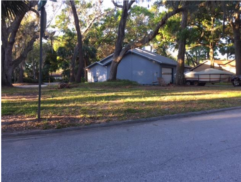
Single-family residence to the southwest of the entrance to the subject site
